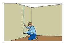
• Using a stud finder to identify studs, mark top and bottom of studs using a pencil.
